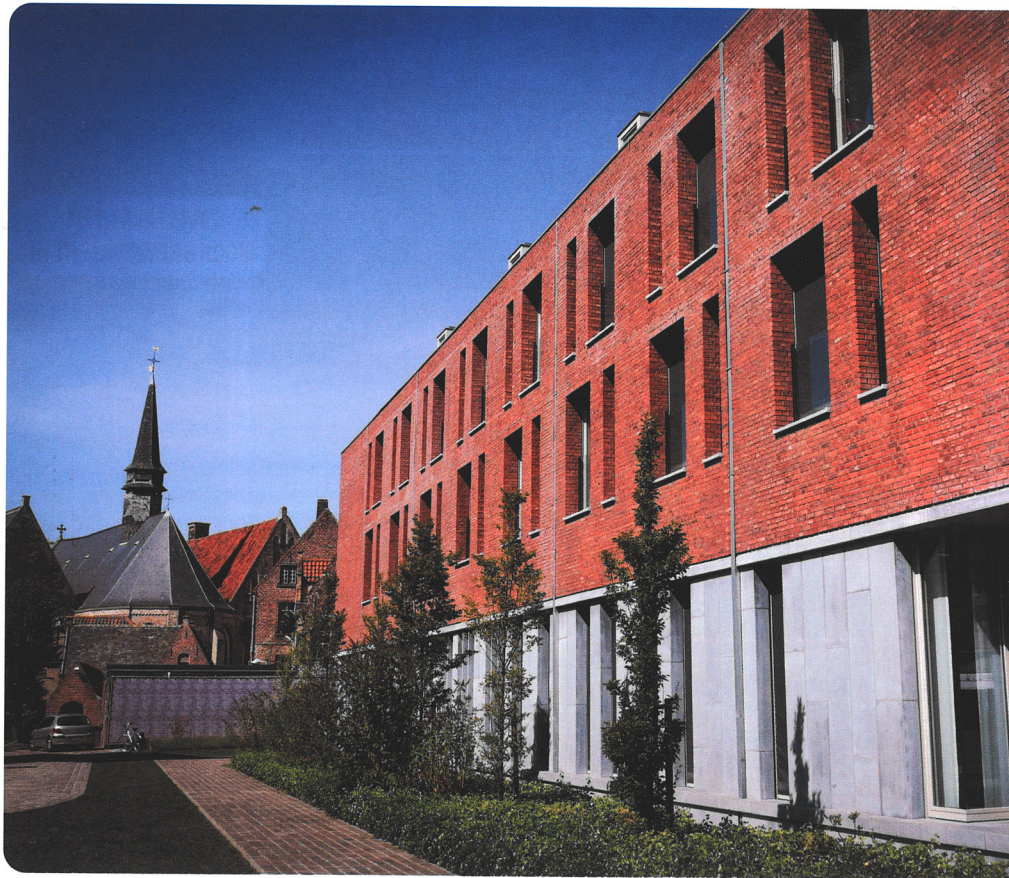
Ter Potterie, in Bruges, Belgium uses an innovative thermal energy system.
