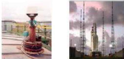
Photo 6: How a petrol tank head and a launch ramp can be protected
