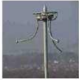
Photos 1 and 2 Radioactive sources Helita (one of the two is positioned below an antenna fitted on the roof of a hospital!)
