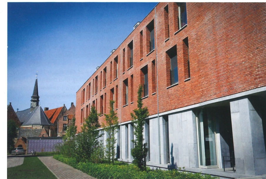
Ter Potterie, in Bruges, Belgium uses an innovative thermal energy system.
